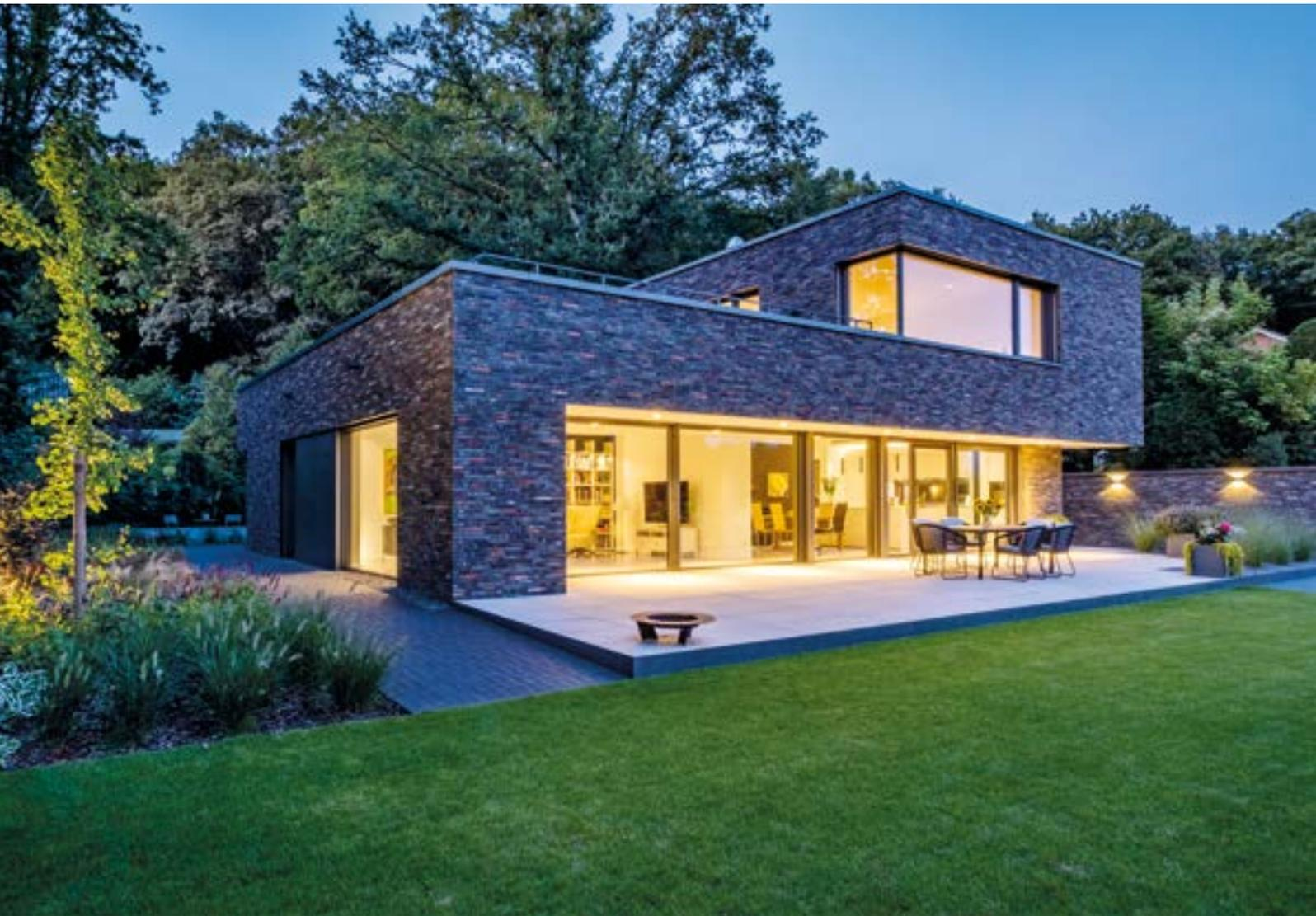
Space is gained with the narrow bricks. Furthermore, a narrower brick means less energy during firing, less clay, and lower resource costs.
